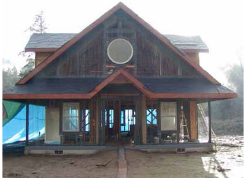
Install mesh before the bales on multiple story homes.
